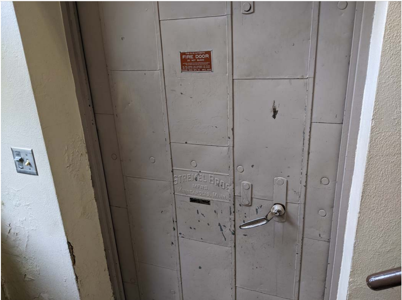
Assumed fire door-Garage
