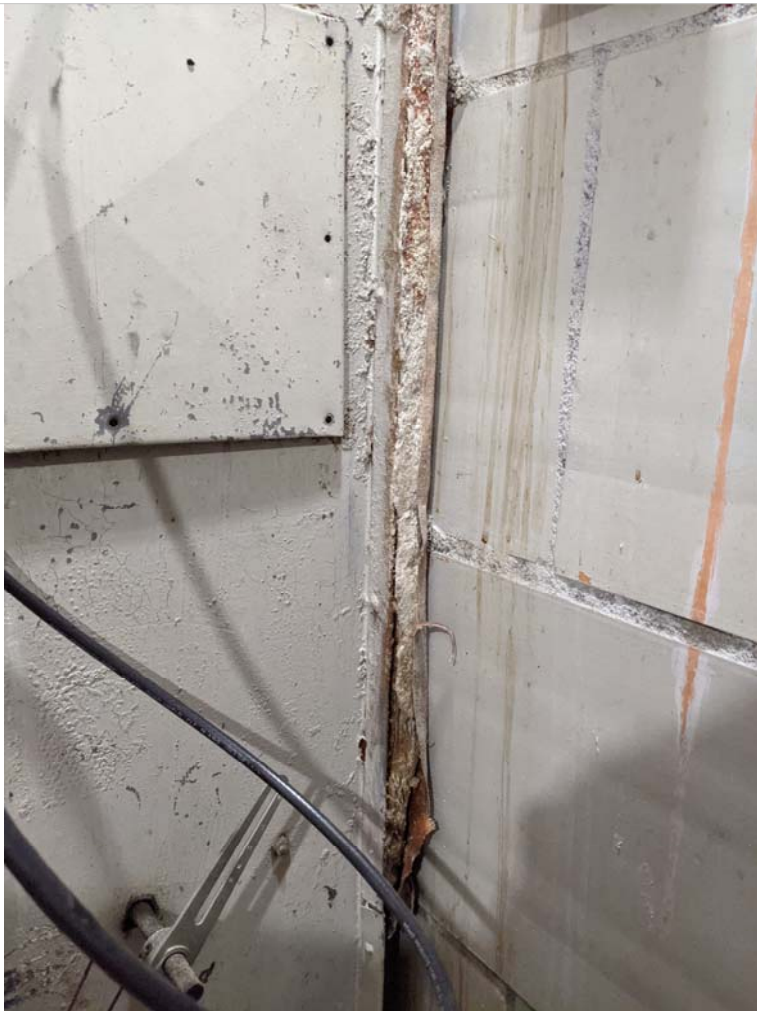
ACM insulation around hvac-equipment room east side
