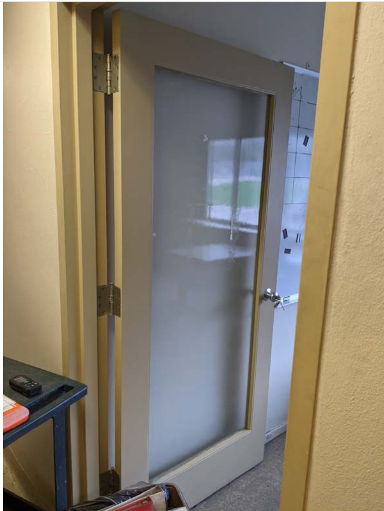
ACM Glazing in door-typical style 1
