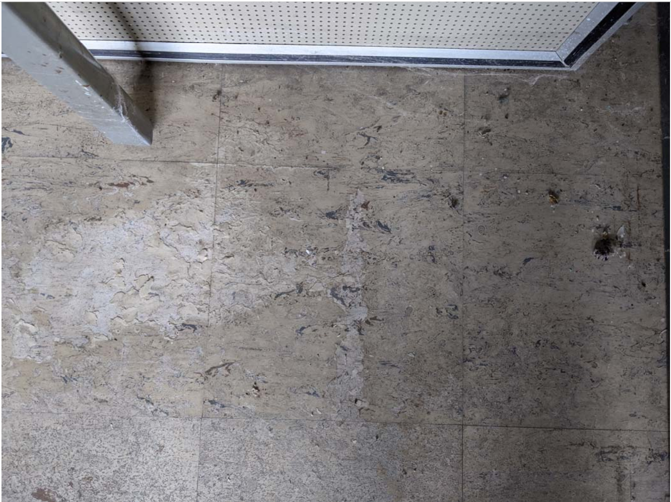
ACM 9 inch floor tile-typical
