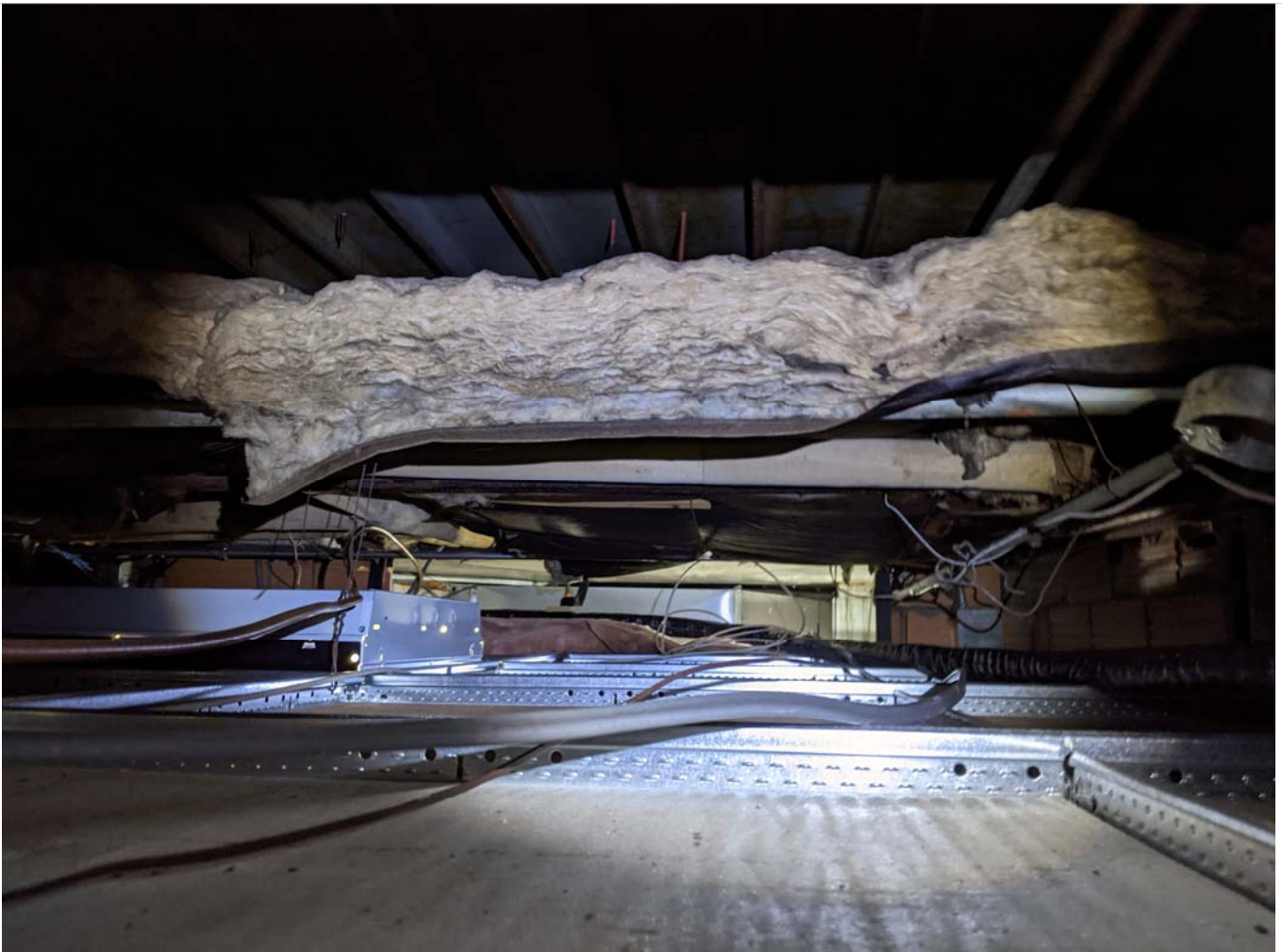
ACM pipe insulation-above ceiling tile-above plaster ceiling-typical
