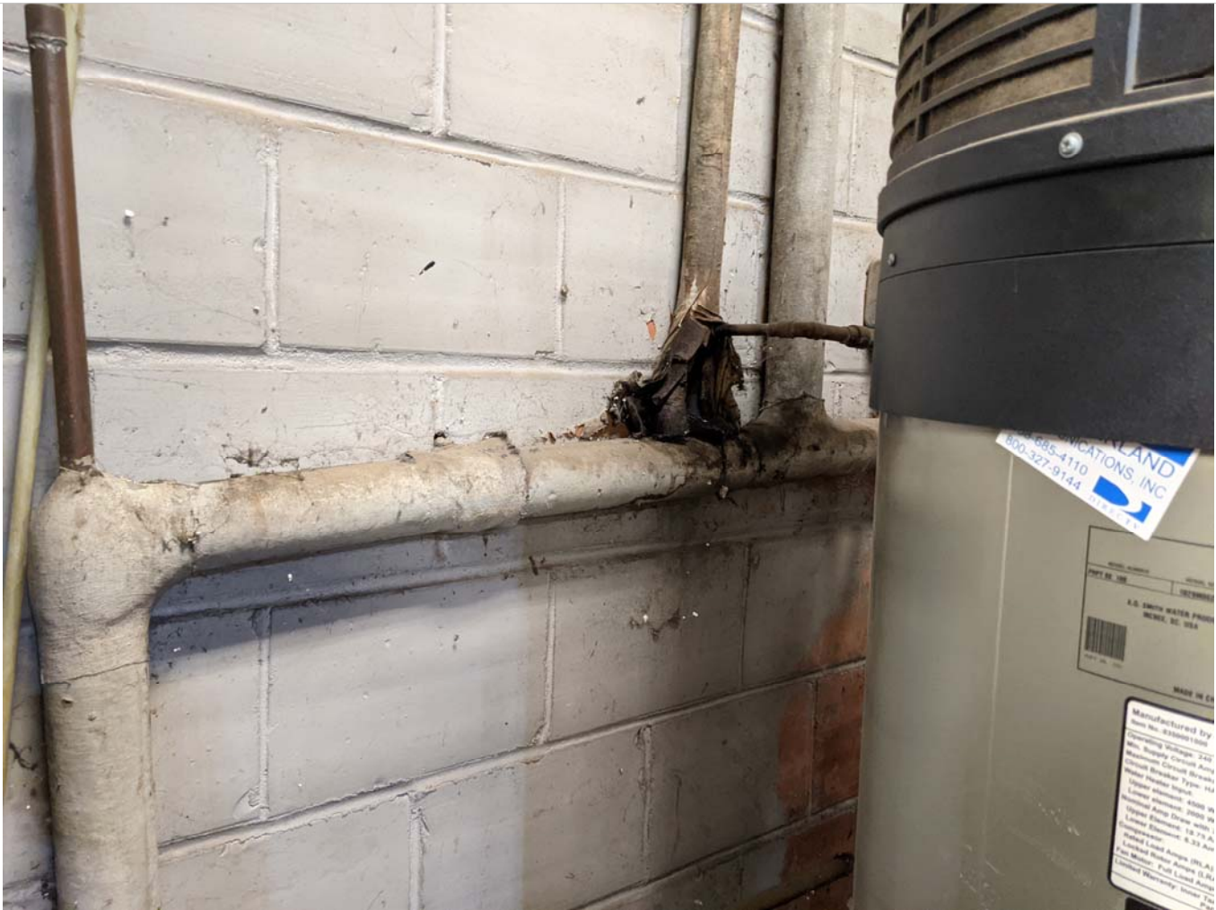
ACM pipe insulation-garage-typical
