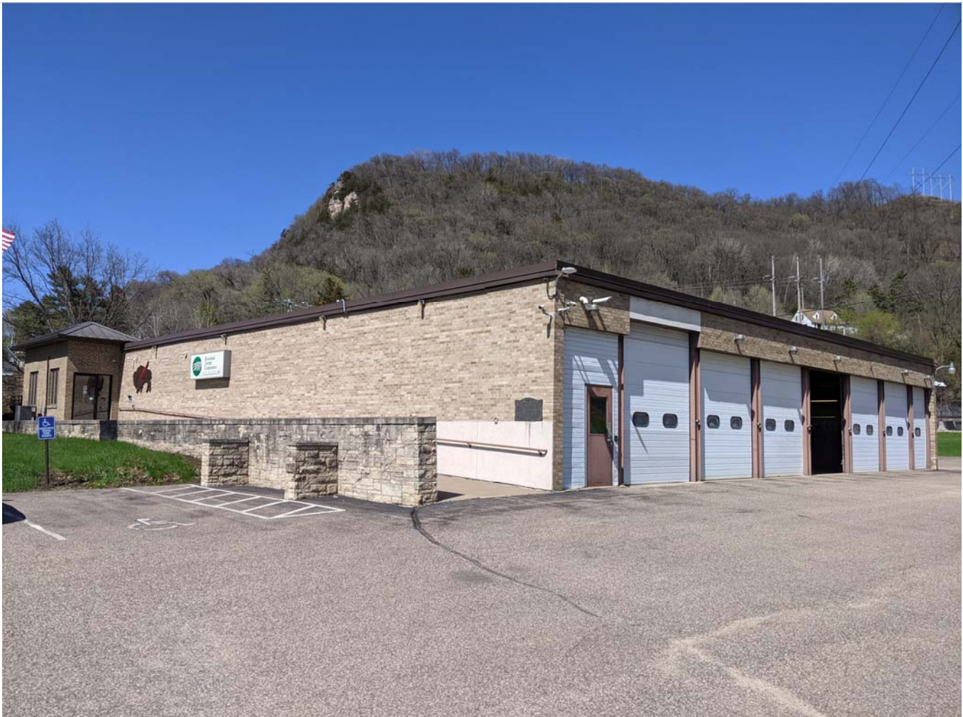
Exterior of Building
