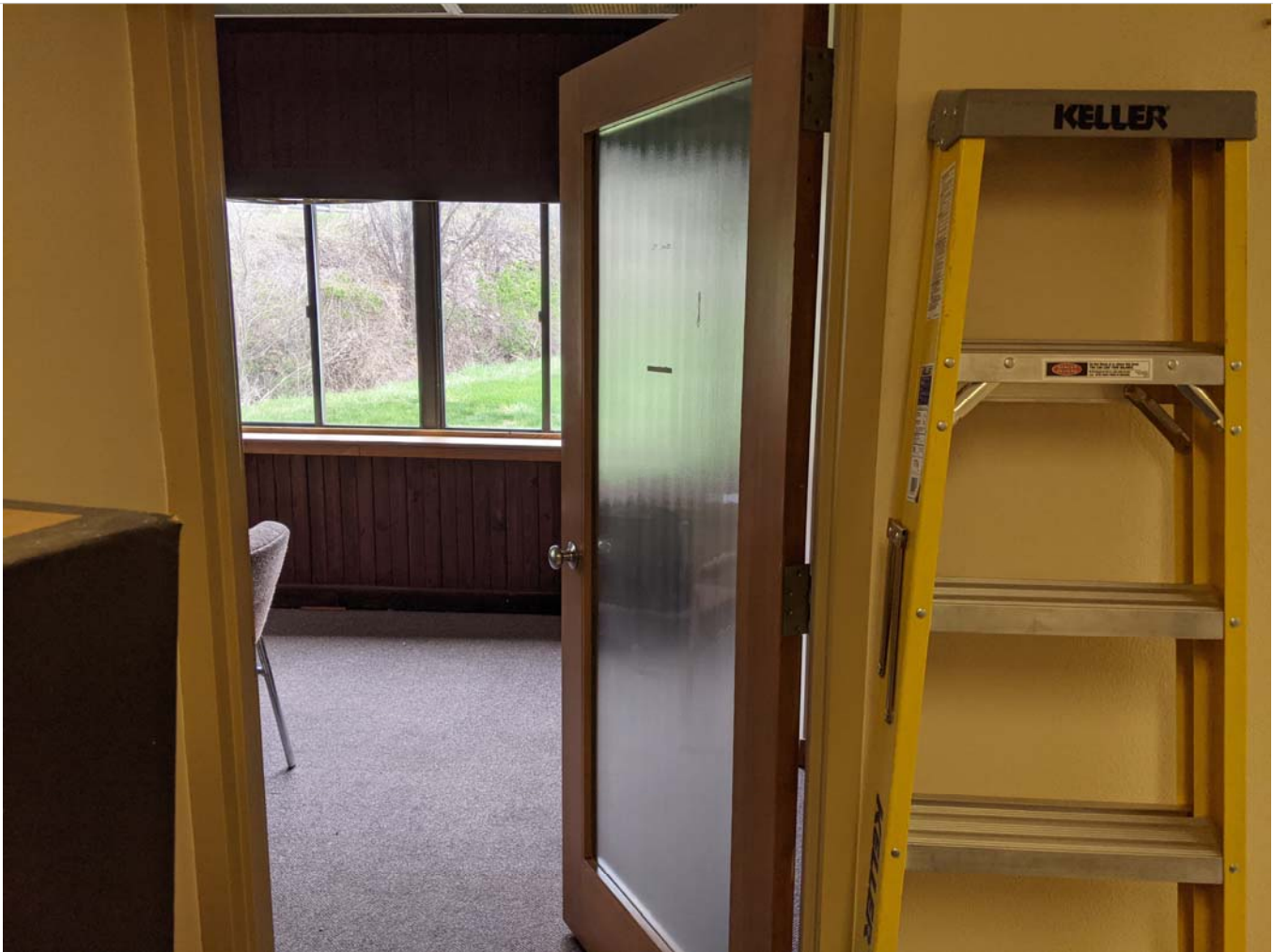
ACM glazing in door-typical style 2
