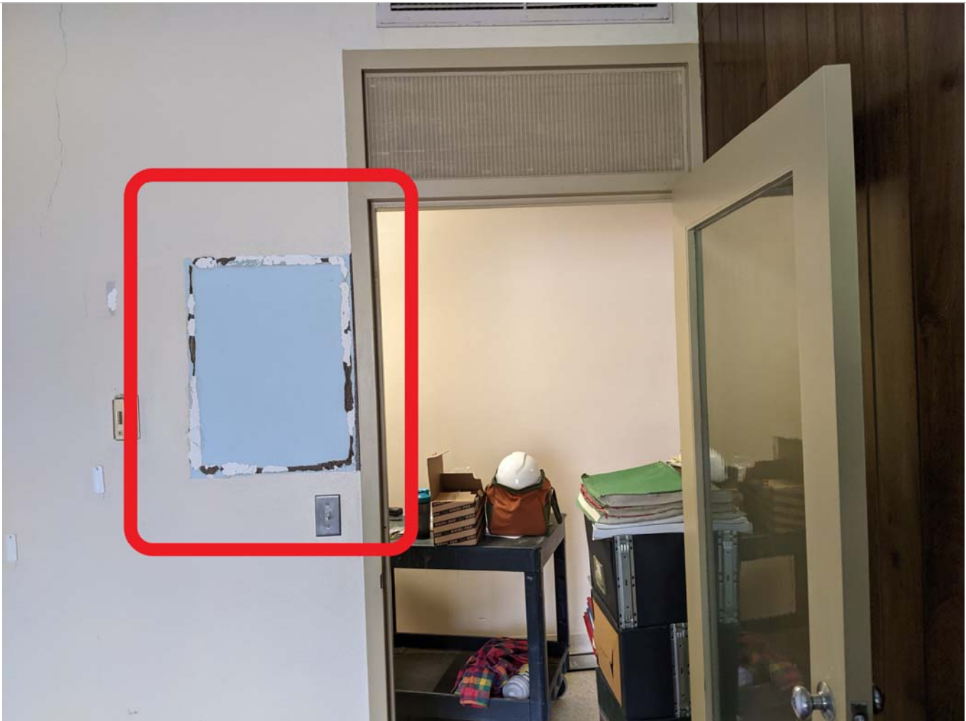
ACM Brown adhesive on wall-RCI Sales, ACM glazing in door
