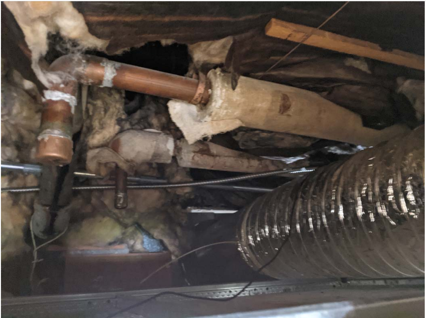
ACM pipe insulation-above ceiling tile-above plaster ceiling-typical
