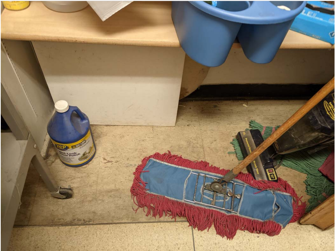
ACM 9 in floor tile-hallway closets-typical
