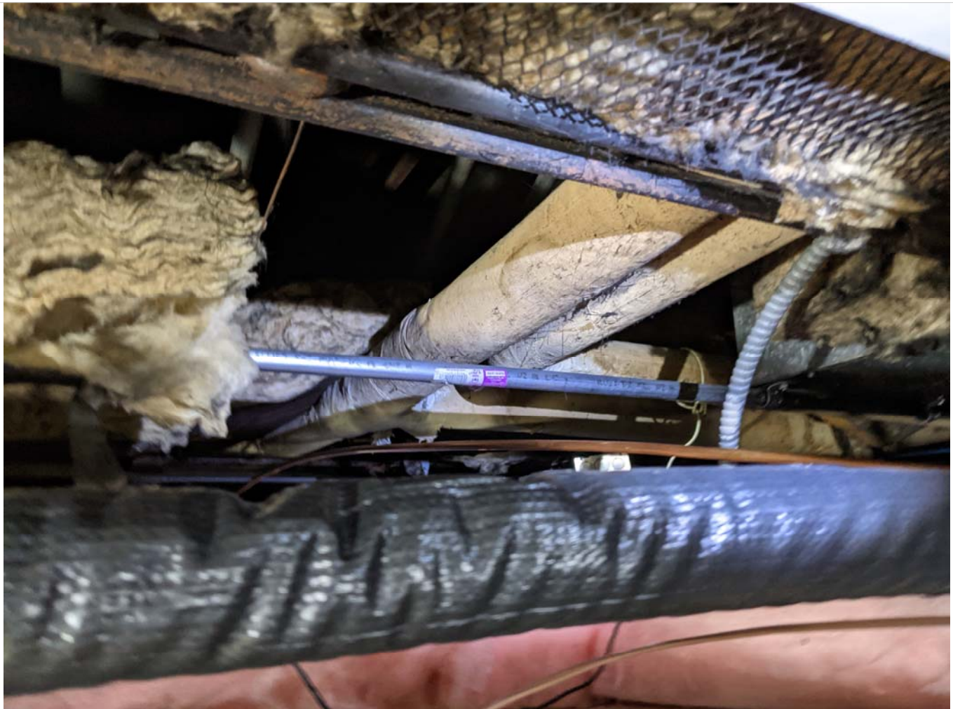
ACM pipe insulation above plaster ceiling-typical
